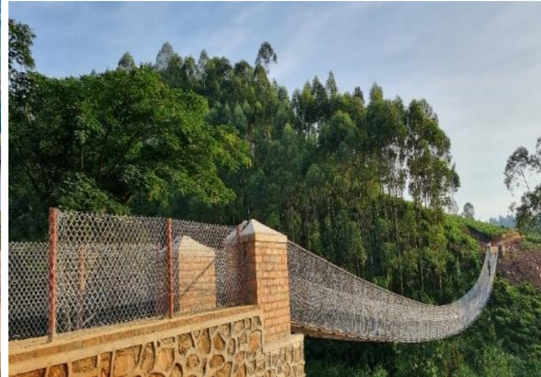
Kishanda-Kisengere Suspended Trail bridge (84m Span), Kanungu district
