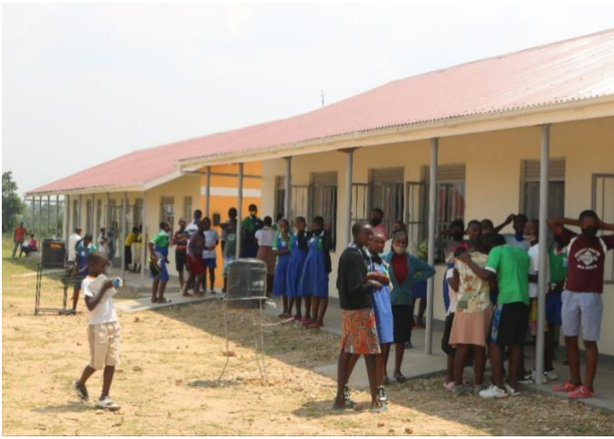
Pupils of Rwamwanja P/school in Kamwenge district in the newly constructed classrooms. The school has a total enrolment of over 1,000 pupils (90% are refugees)
