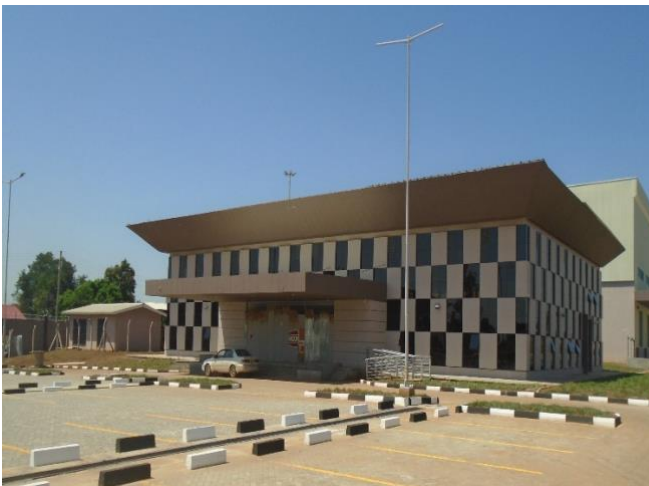
Construction progress of the Gulu Logistics Hub administration block and the container freight station.
