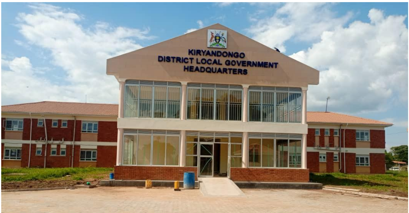
Kiryandongo District headquarters constructed under the project
