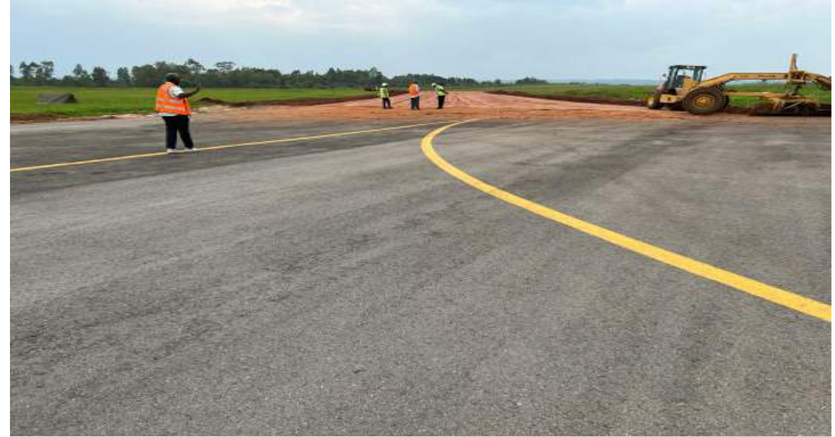
Arua airfield works
