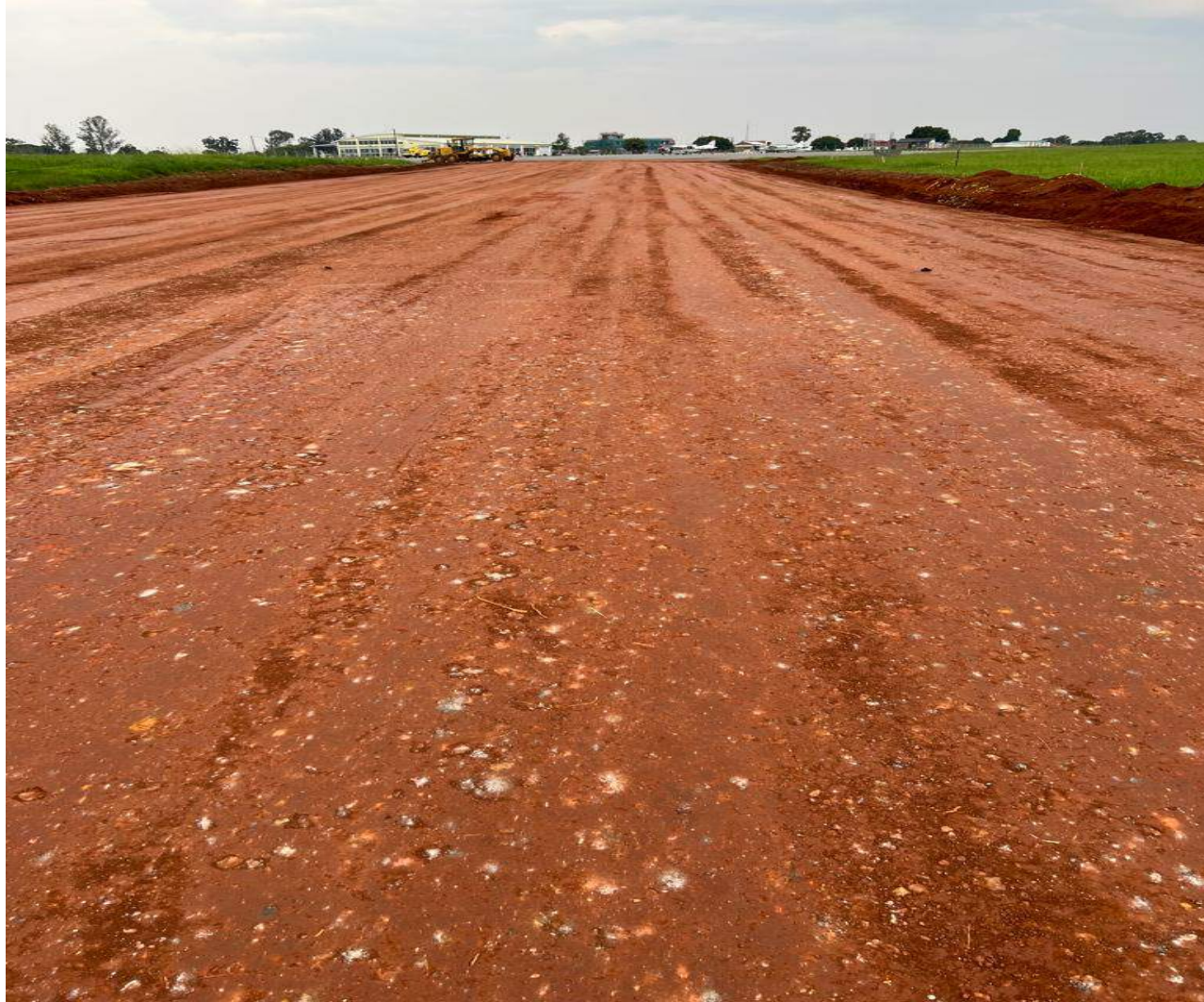
Arua airfield taxiways re-construction
