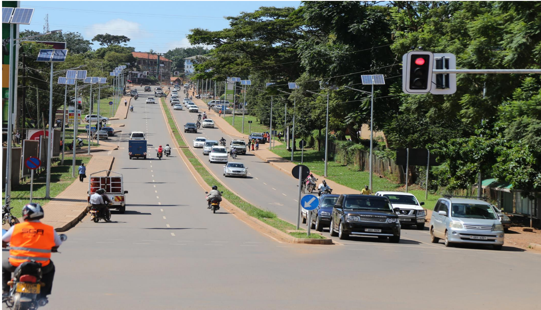
Kira road Junction reconfigured and signalised under the KIIDP II project
