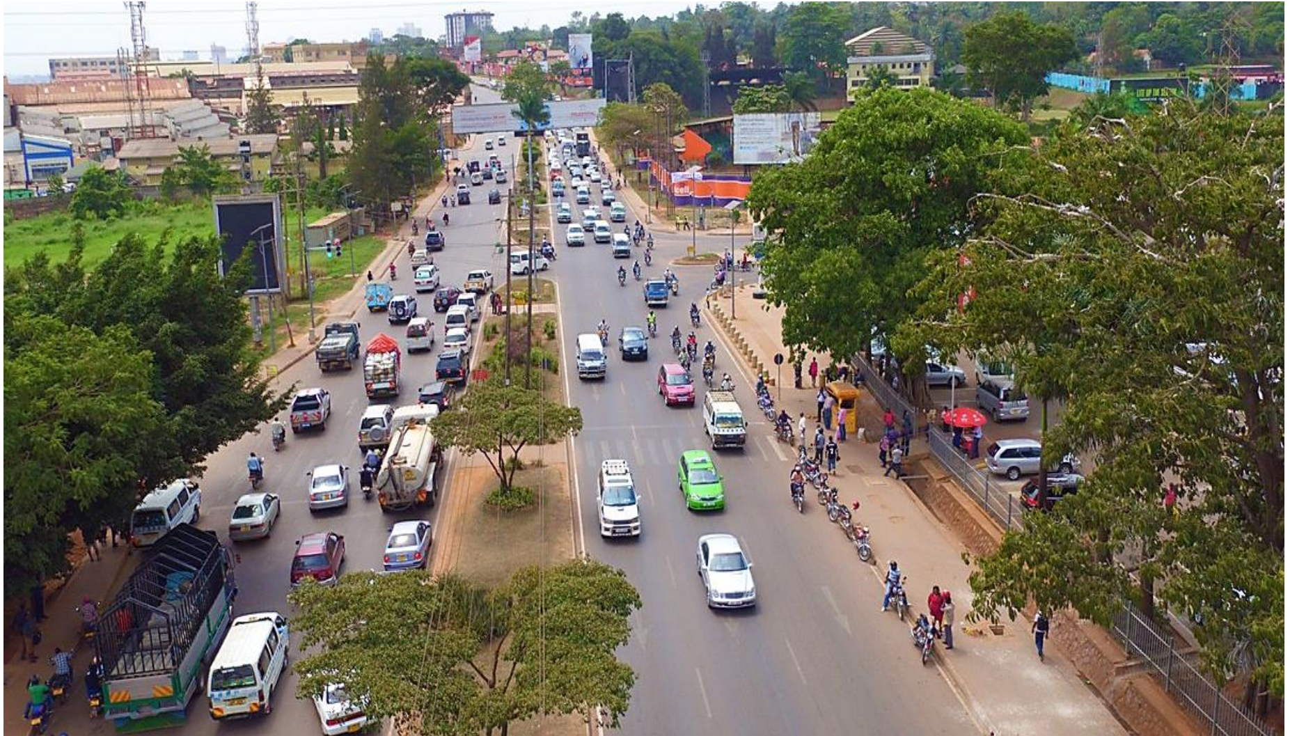
Jinja road (Lugogo) Junction reconfigured and signalised with support from JICA
