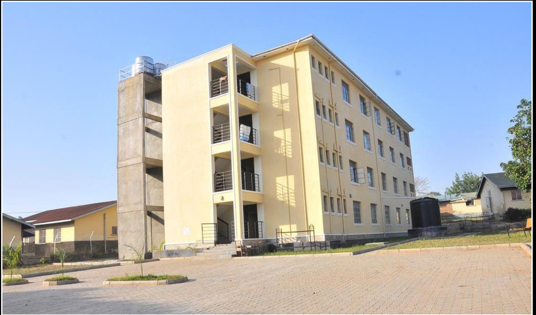
A 240-bed capacity Girls' Dormitory completed and commissioned on 18 th Dec. 2022 at Arua School of Comprehensive Nursing and Midwifery, Arua district.
