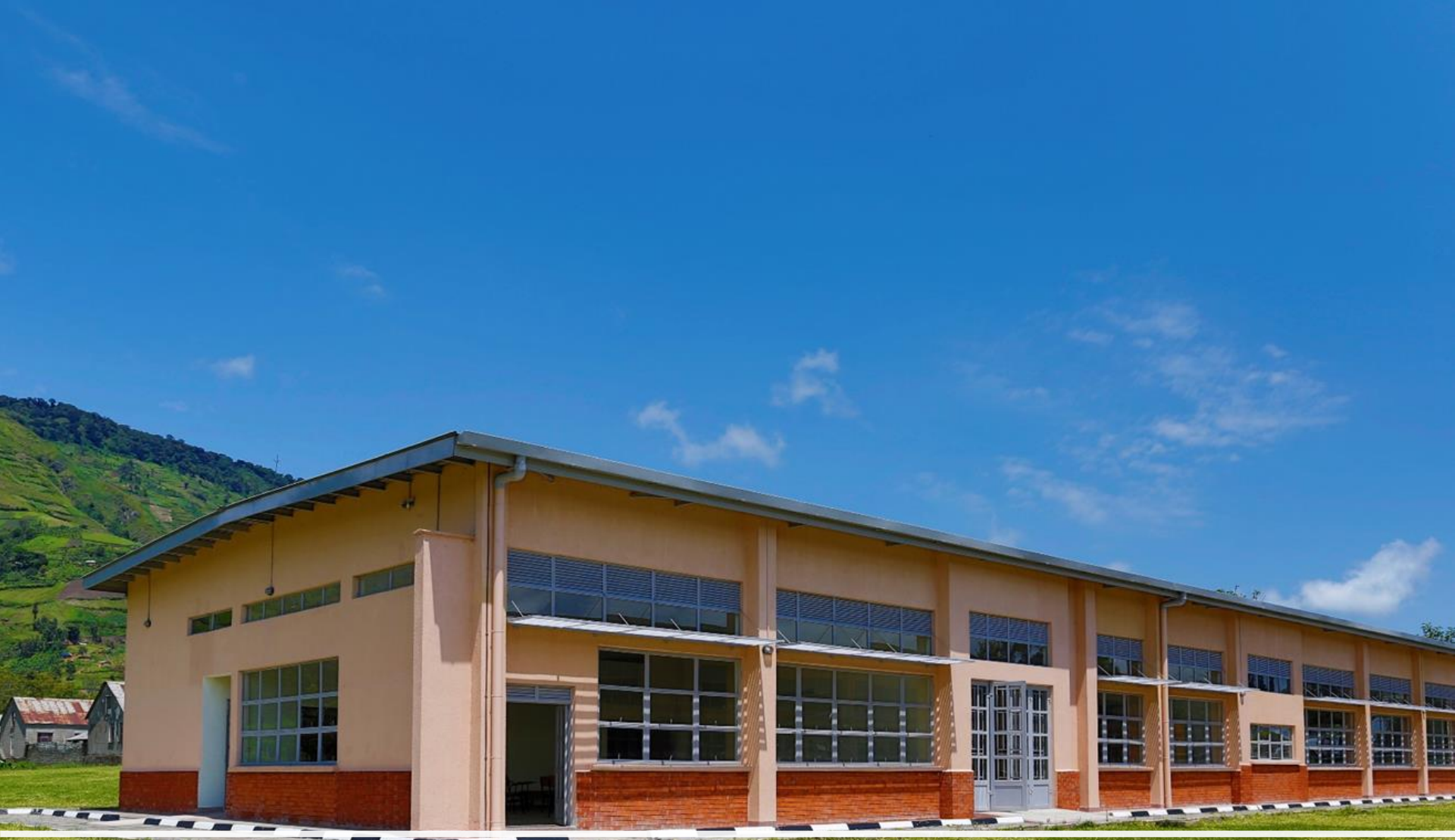
A newly built Welding and metal fabrication workshop at UTC Kichwamba, Kabarole district.
