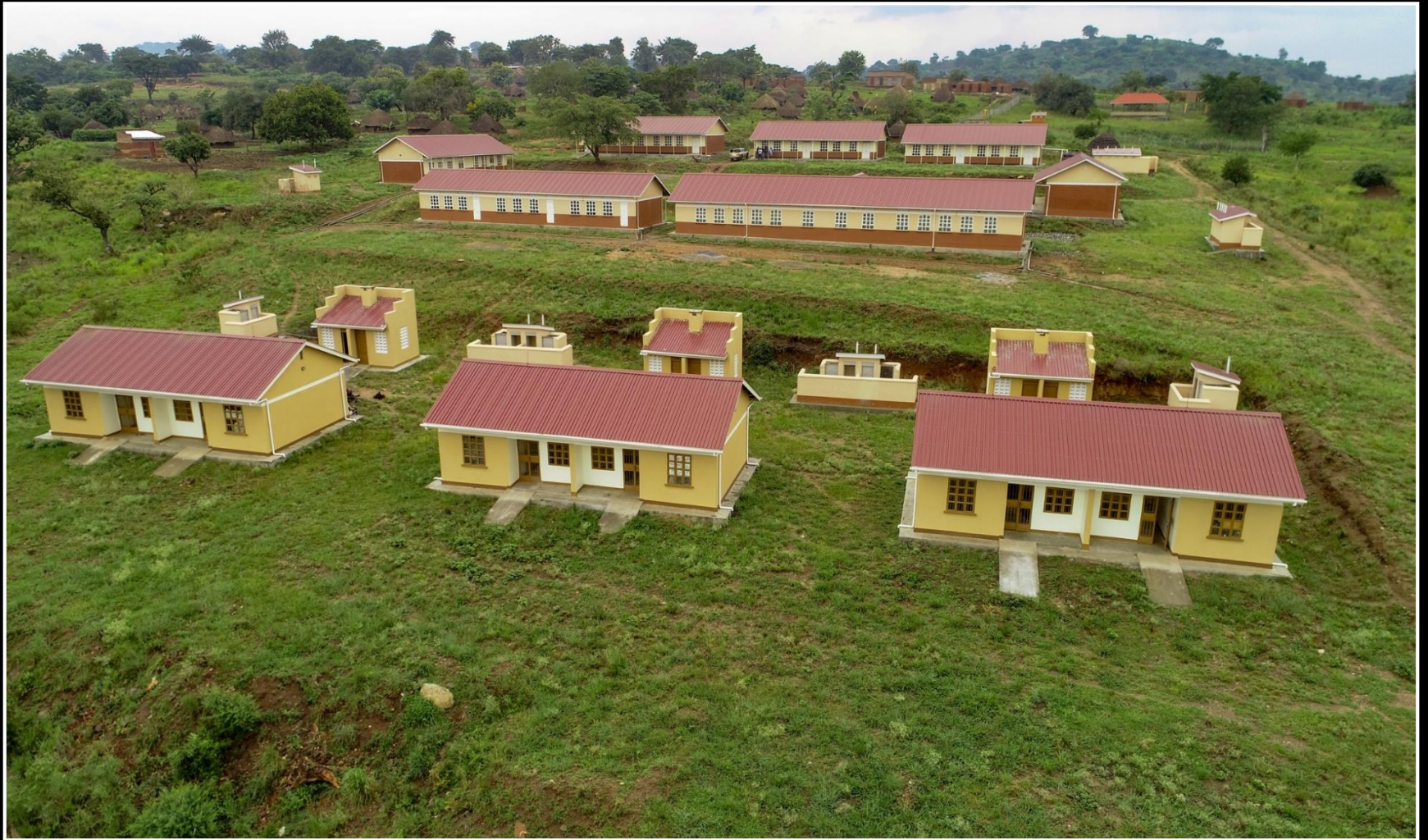
Atego Seed Secondary School, Nebbi District, constructed under UgIFT-1
