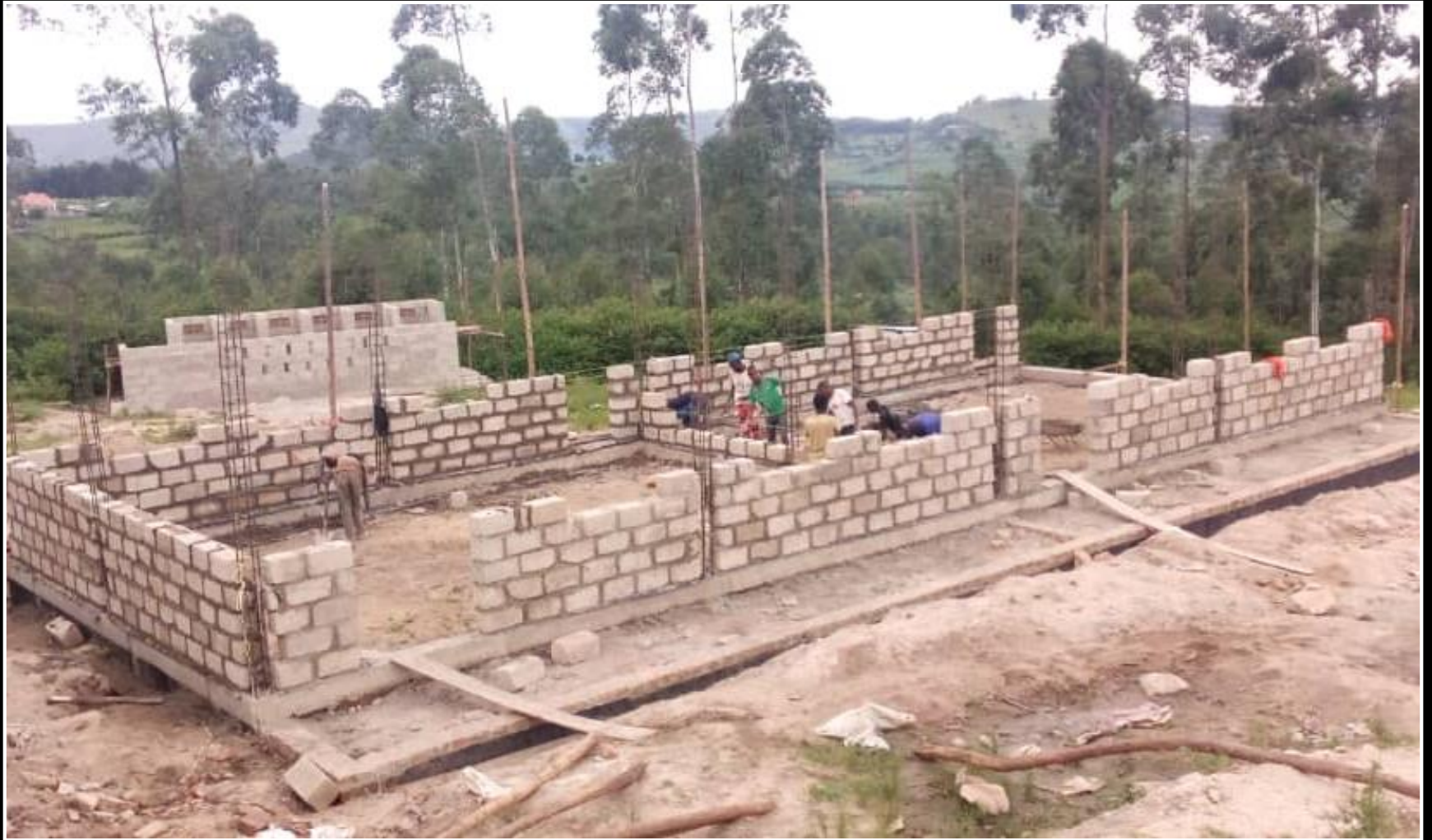
Construction Work at Nyabihoko Seed Secondary School, Ntungamo District under UgIFT-Phase 2.
